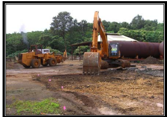
- Site Prep Prior to Dioxin Soil Sampling -
