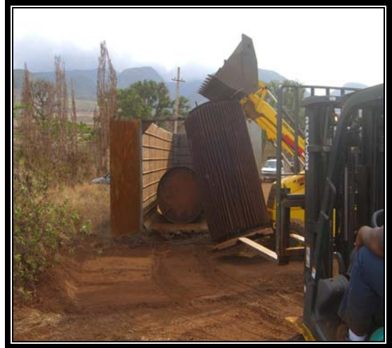
- Transformer Carcass Disposal -
