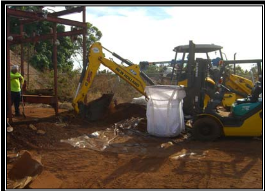
- PCB-Contaminated Soil Removal -
